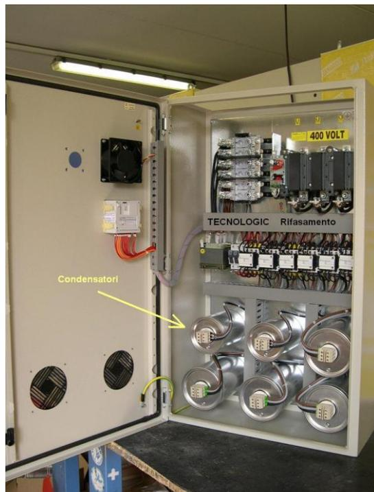
Figure 121: capacitors installed in the electrical panel
