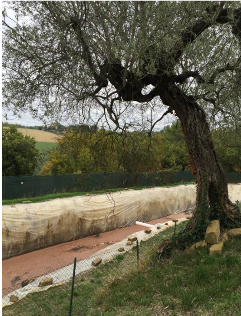
Εικόνα 133: basin for the storage of vegetation water
